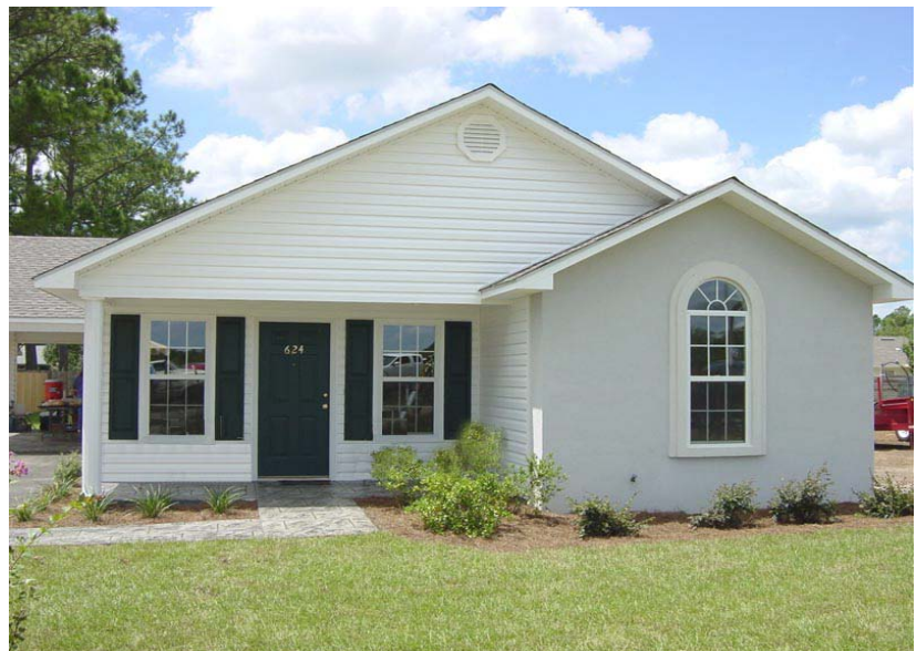
This EasyLiving Home offers a step free entrance Photo credit: EasyLiving Home cm
