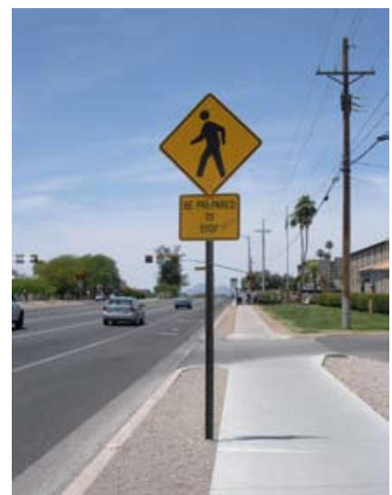
BE PREPARED TO STOP pedestrian sign prior to the HAWK installation.
