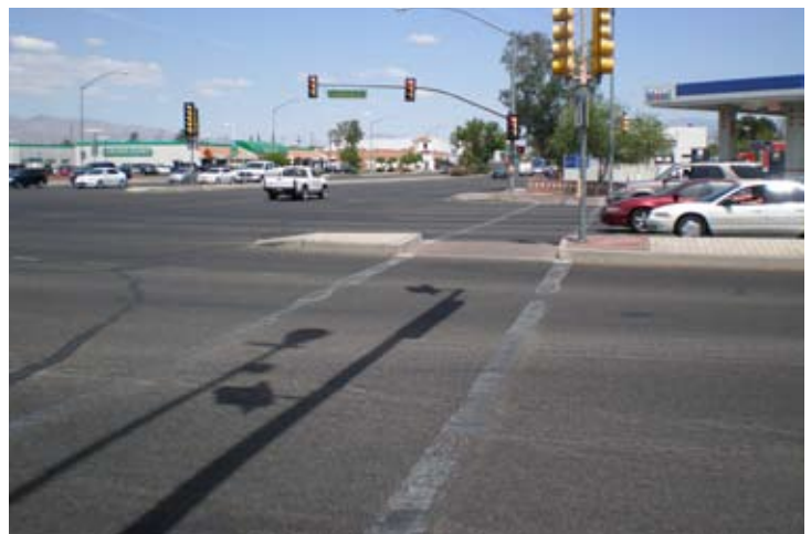
A cut-through median at the intersection.
