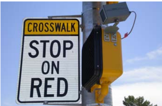
A microwave detector mounted on a pedestrian indication at a Puffin Signal.
