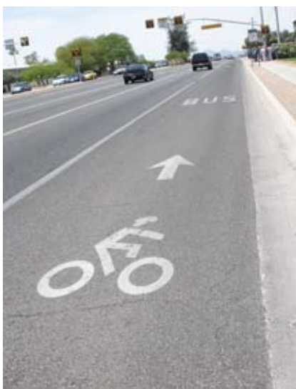
A marked BUS and BICYCLE ONLY lane in the right-curb lane approaching the mid-block HAWK signal.
